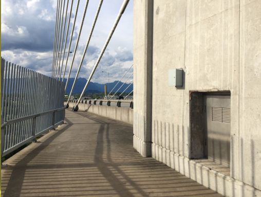
Door with bridge view
