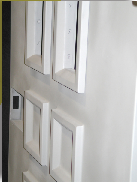
Showing the projection of the raised panels
